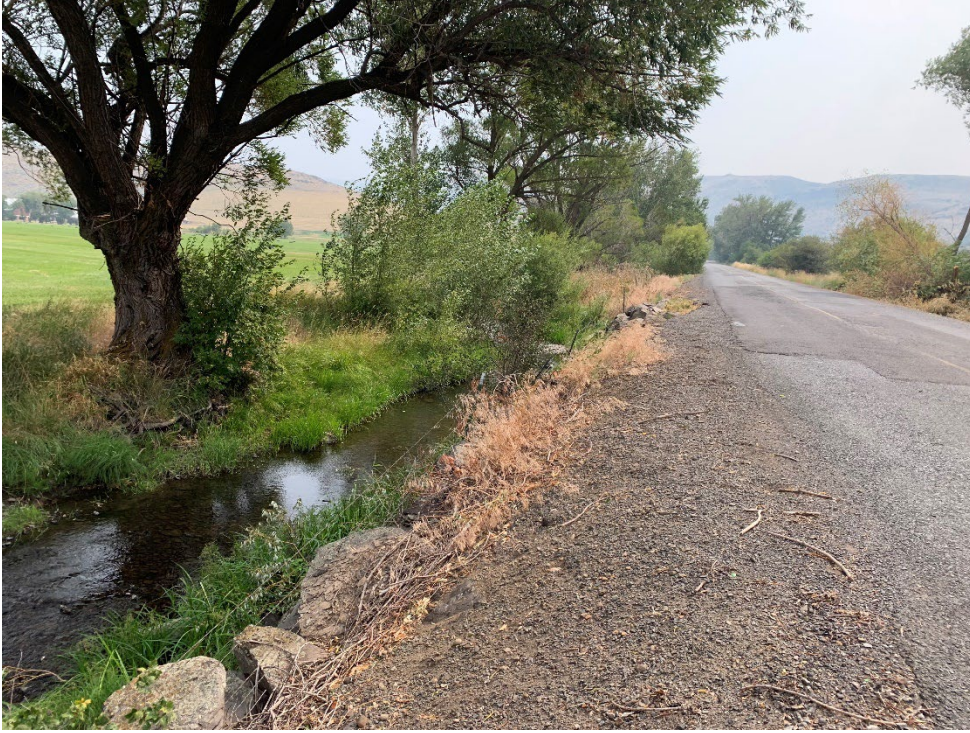
Figure 19 - Little Creek to the east of Kofford Road.
